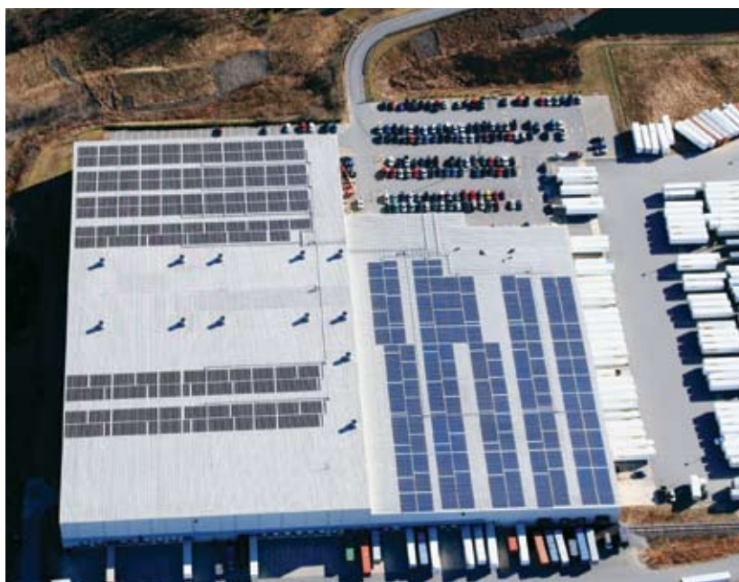
DELIVER US In 2007, when SunEdison built this solar array on the roof of Staples’ Killingly, Connecticut, distribution center, it was New England’s largest—the size of 1.5 football fields.
